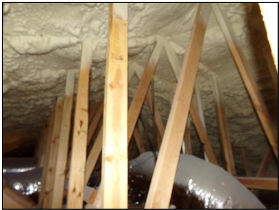
3.7 Item 2(Picture) Polyurethane Foam - Attic 2
