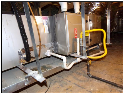
8.0 Item 7(Picture) Attic Located Air Handler
