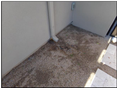
3.4 Item 1(Picture) Splash Guard Needed 1
