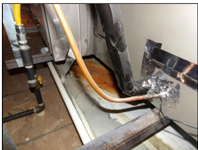
8.5 Item 1(Picture) Rusted Condensate Pan
