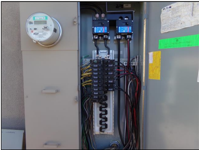
6.1 Item 2(Picture) Main Electrical Panel - Interior
