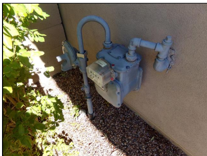
5.6 Item 1(Picture) Main Gas Valve and Meter
