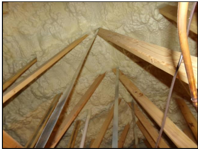
3.7 Item 1(Picture) Polyurethane Foam - Attic 1
