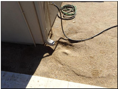
3.4 Item 2(Picture) Splash Guard Needed 1
