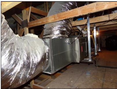
8.0 Item 8(Picture) Attic Located Air Handler 2
